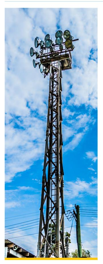
68/2 (half the pitch width) + 5m (Runoff) + Foundation (1m) = 40m.  $40m \times 0.36 = 14.4m$ .
