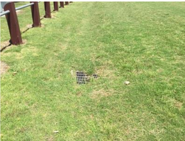
Drainage system present, but dysfunctional
