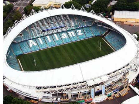
Allianz Stadium Upgrades
