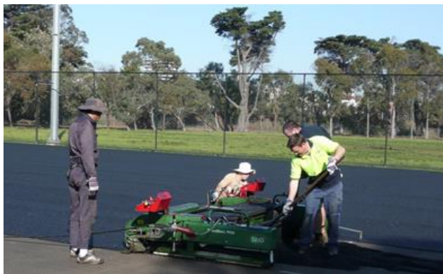
Photo 28: Insitu Shockpad being laid (Source: Polytan)
