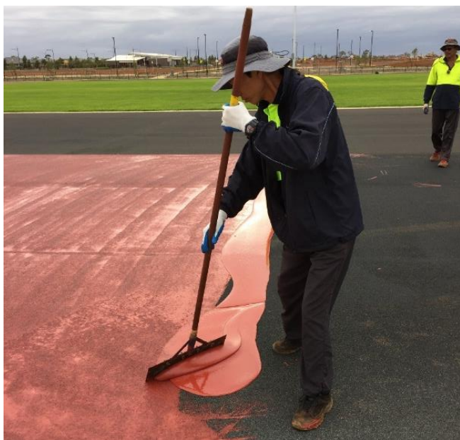
Photo 32: Application of wearing layer over rubber base mat
