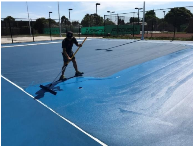
Photo 35: Application of acrylic system
