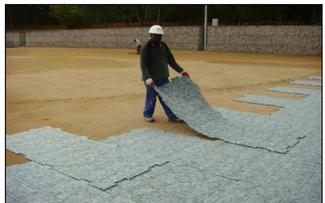
Photo 27: Prefabricated Shockpad being laid (Source: TEAM Sports)
