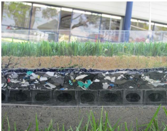
Photo 29: Example of horizontal drainage cell under shockpad (Source: Wayne Stuart - City of Swan, WA)
