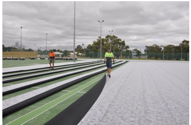
Photo 36: Installation of prefabricated mat system
