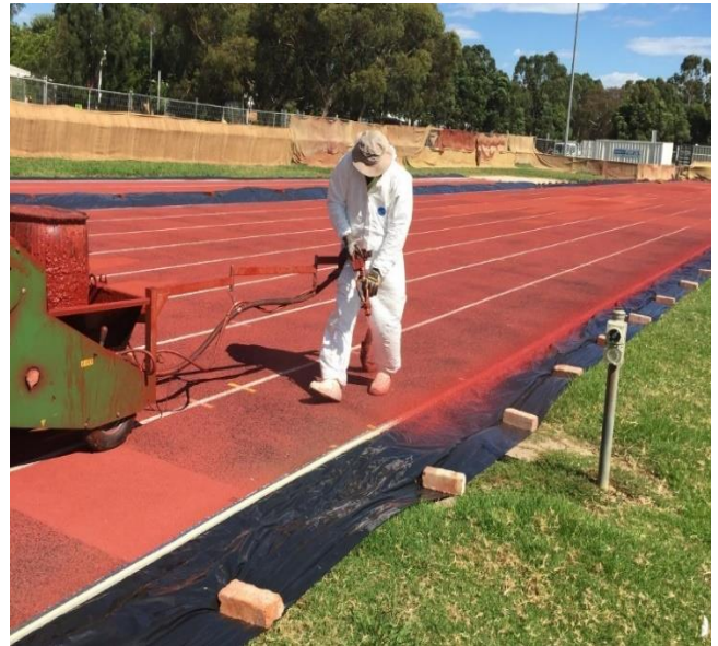
Photo 31: Application of spray coat
