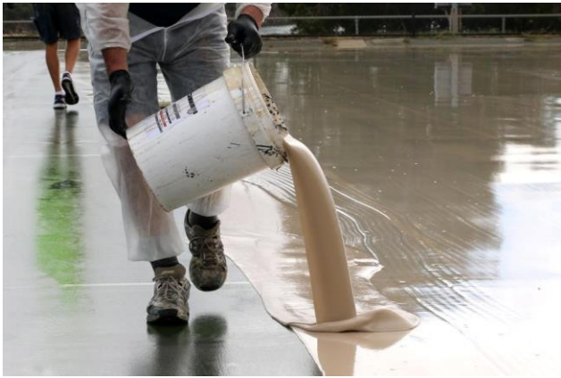
Photo 37: Application of gel system
