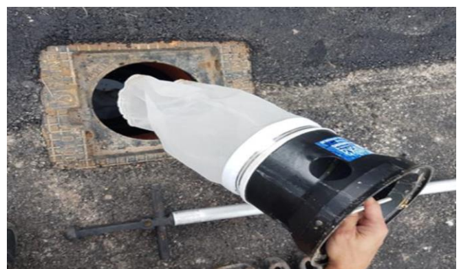
Photo 16: Containment strategy example 3: Drains fitted with filter
