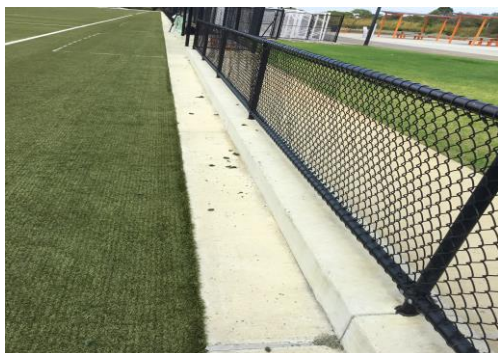
Photo 14: Containment strategy example 1: Curb to reduce the infill being dispersed outside of the field of play
