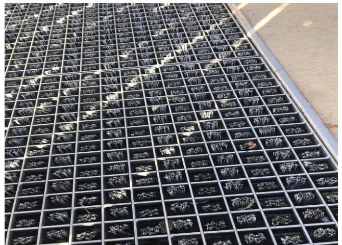
Photo 15: Containment strategy example 2: Pedestrian gates mats that capture the infill
