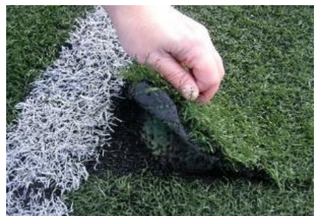
Photo 12: Example of seam becoming undone and can cause a trip hazard (Source: Alastair Cox Associates)
