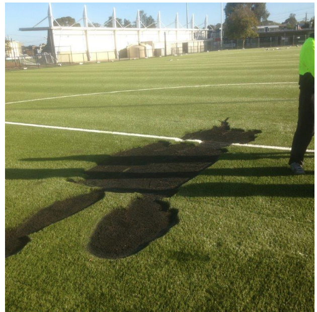
Photo 28: Vandalism can entail a whole section being cut out and replaced
