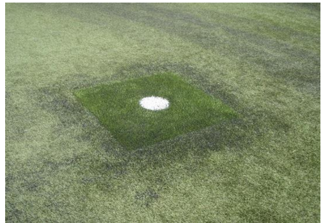
Photo 31: Replacement penalty spot due to excessive wear
