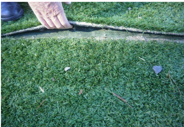
Photo 13: Seam has come apart, needs specialist to sew and or re-glue
