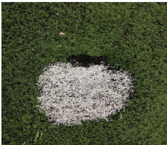
Photo 9: Heavy wear area of penalty spot that needs replacing as dangerous trip hazard (Source: Smart Connection Consultancy)
